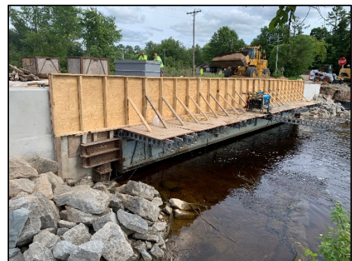
CTH M Bridge under construction in Neopit
