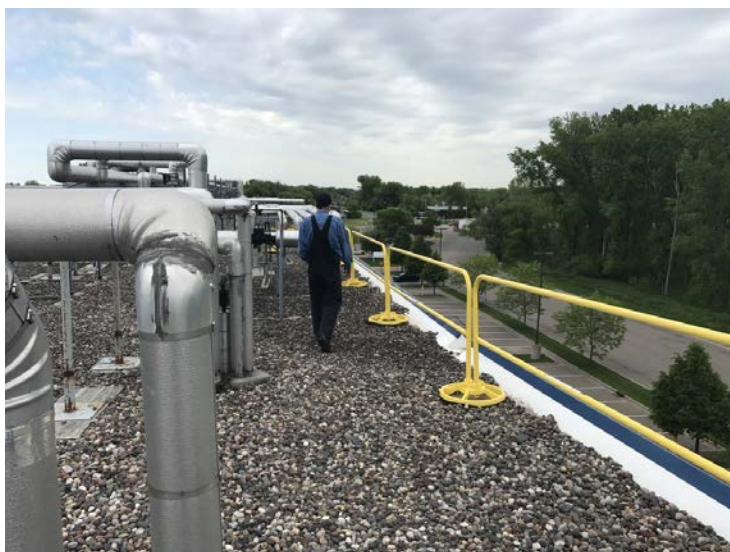
Passive System - Guardrails
