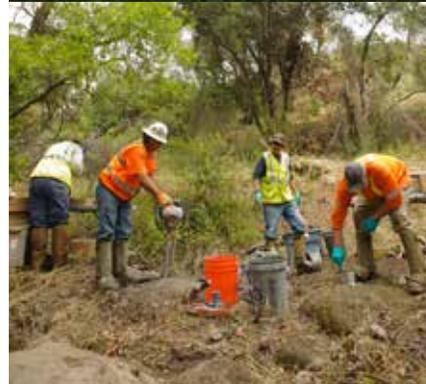
**Left:** A team installs groundwater monitoring wells as part of Boeing's seeps and springs investigation. Boeing has a network of more than 450 wells to monitor legacy contamination in the groundwater below the Santa Susana property. (Boeing photo)
